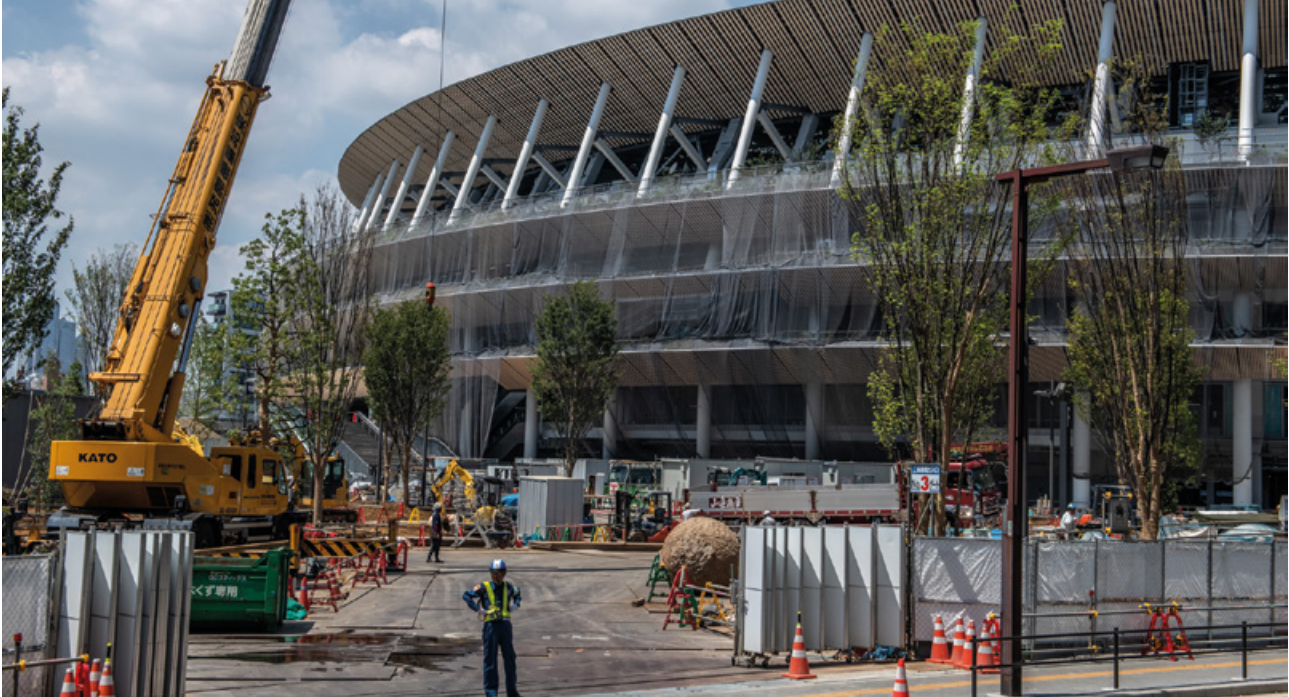
Work continues on the new National Stadium, the main stadium for the upcoming Tokyo 2020 Olympic and Paralympic Games (Carl Court/Getty Images)
