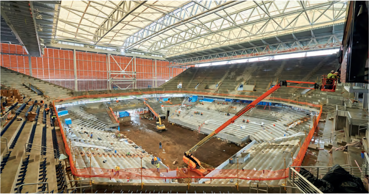
The new Louis Armstrong Stadium under construction (US Tennis Association)
